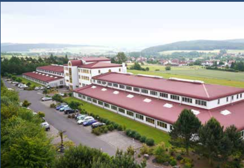
Plant in Eichenzell 36124 Eichenzell, Hesse Total area: approx. 30,000 m 2
